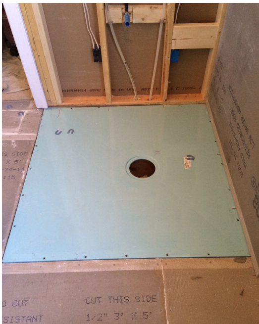
Classic shower base installed on joists.
